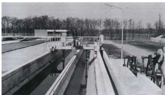
Figure 2.7 - Rectangular horizontal flow grit chamber
