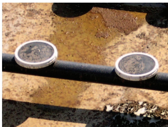
Figure 3.13 - distribution of the elements over the bottom creates spiral flows (whirlpools); a. spiral flow; b. ridge and furrow; c. bottom aeration
